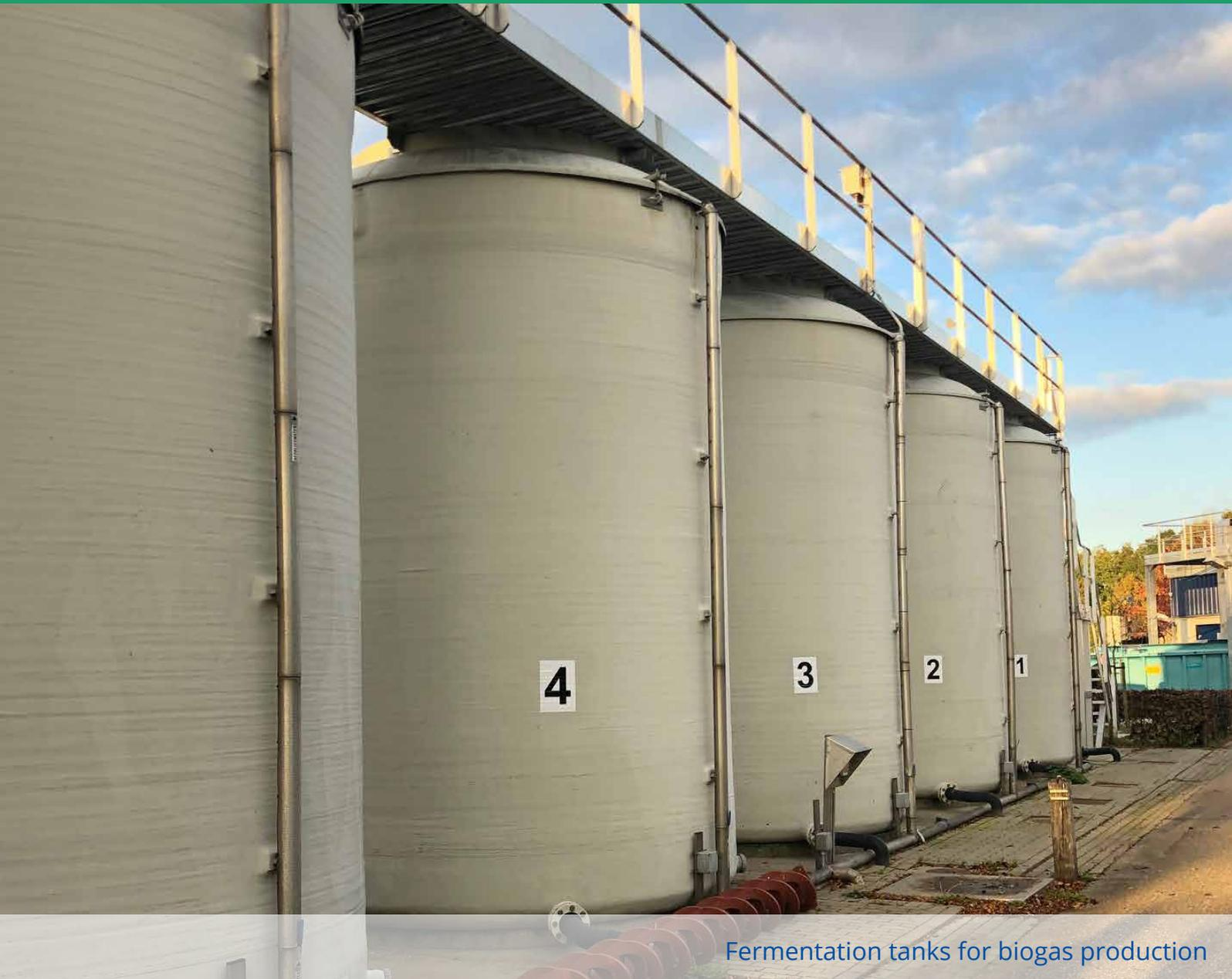
Fermentation tanks for biogas production
