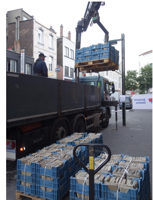
Dismantling and reclamation of construction elements
