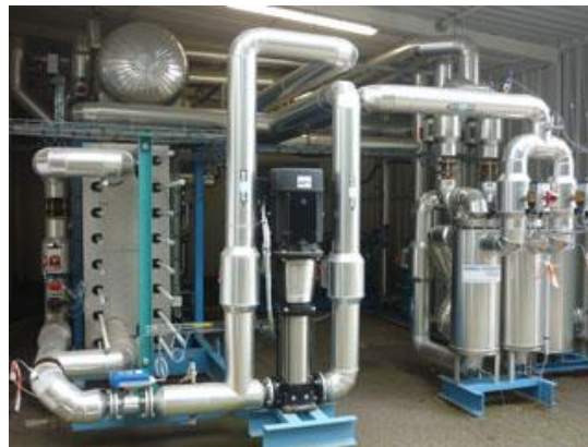
Figure 24: Ice slurry generator system [36]
