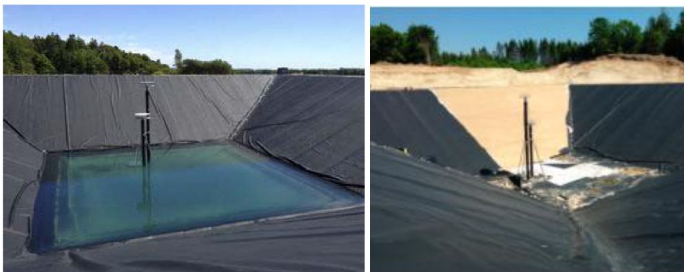
Figure 19 : Picture of Dronninglund Pit Storage under construction [33]
