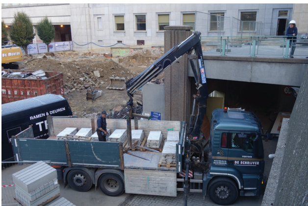
Reclamation of marble floor slabs, from dismantling to resale point (marble from Brussels North Station, by Rotor DC).
